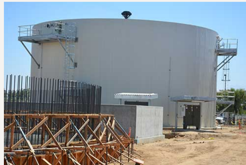
The $30 million digester works at 130 degrees to convert food waste and other organic materials into fertilizer and fuel.
