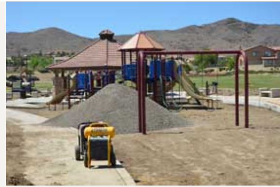
The play area at Monument Ranch Park also is undergoing significant renovations with a new “soft-fall” surface.
