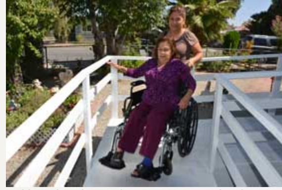
Perris resident Maria Teresa Montes, 80, and her daughter, Elsie Ramirez, make their way along a ramp installed as part of the City of Perris Senior Home Repair Program.
