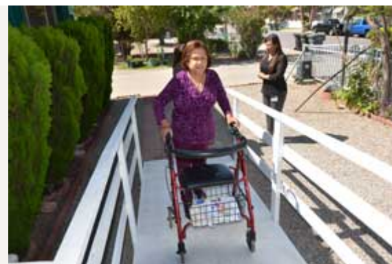
Perris resident Maria Teresa Montes, 80, walks up a ramp at her residence that was installed as part of the Senior Home Repair Program.
