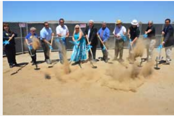
Members of the Perris City Council join other dignitaries in throwing the ceremonial first-shovels of dirt at the ground-breaking of the new Walmart Super Center in Perris.
