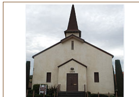
Lewis Hunter purchased this building for $2,000 and moved it to the site of Woodcrest Community Church on Van Buren Boulevard in Riverside.
