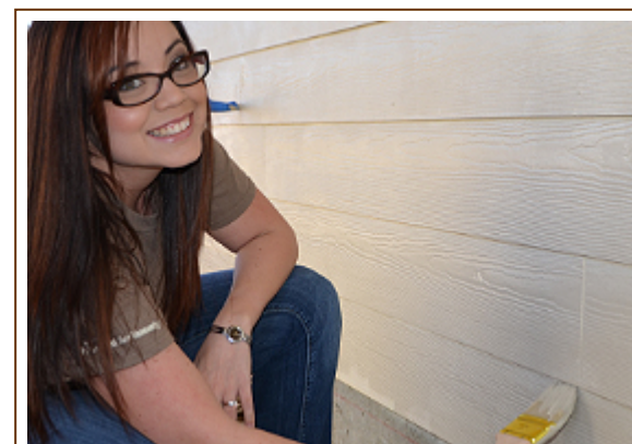
Perris City employee Adrienne Morales rolls paint at the Gomez residence on Eleventh Street in the City's historical Downtown area.
