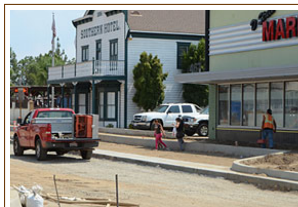
Construction along D Street includes new street work, sidewalks and landscaping.
