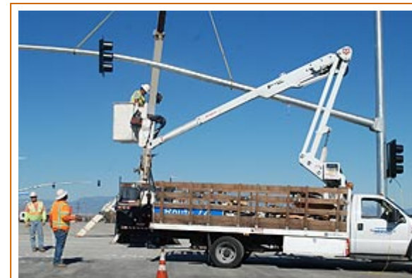
Recent construction work includes putting up traffic signals.
