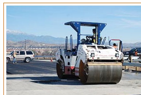
Construction crews blacktop the new Highway 74 (Fourth Street) Bridge over Interstate 215.
