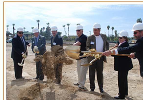
City officials toss the first ceremonial shovels of dirt at the ground-breaking of the Perris Station Apartments Wednesday afternoon.
