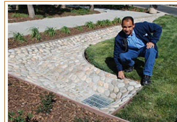
Perris Public Works employee Arturo Garcia inspects a recently completed storm drain at the City Hall Campus, part of the recently completed beautification project..
