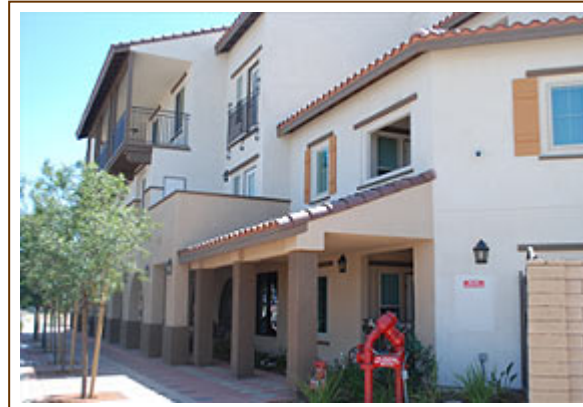
An exterior view of the Mercado Apartments at 832 D Street.
