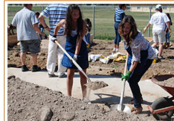
Marina Salcido, 10, and Lana Erickson, 12, shovel dirt to prepare the garden.
