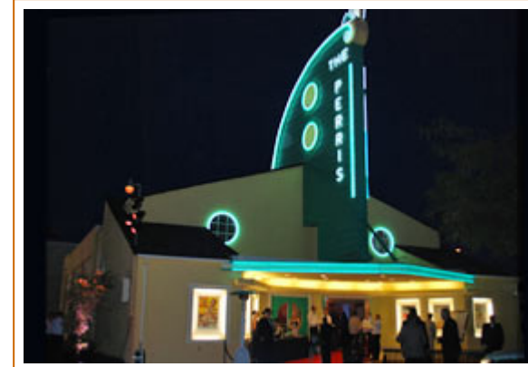
The Perris Theatre after the first renovation.
