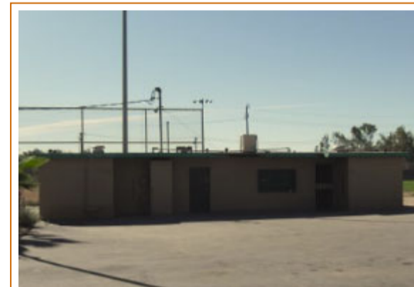
Before image of the concessions building at Bob Long Memorial Park in Perris.
