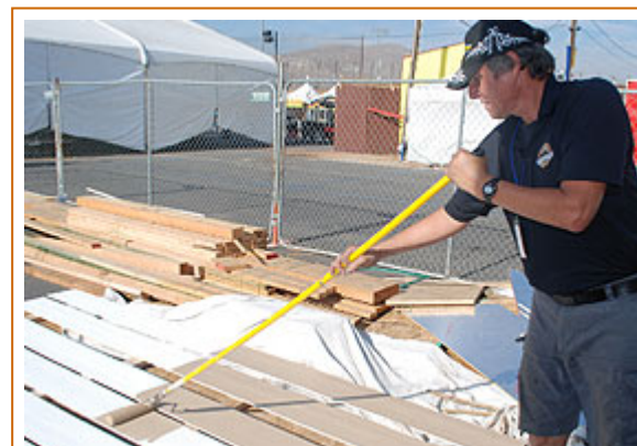
Perris City Councilman Mark Yarbrough rolls a coat of paint on exterior siding during a work shift at the site.
