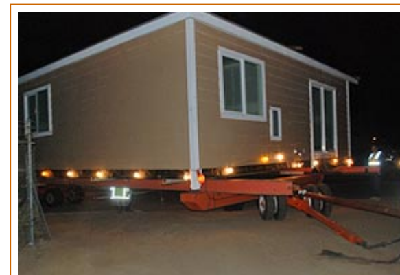
The home is unhitched as it moves into its permanent location on East Second Street in Downtown Perris.
