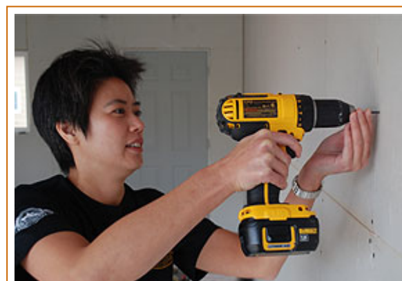
Misty Cheng, Perris' Interim Finance Director, installs a section of drywall.
