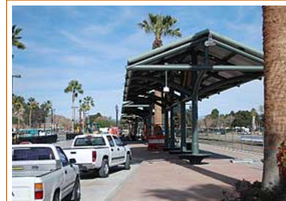
Work crews are finishing up the last bit of work at the Perris Station Transit Center on C Street. The Center features five bus bays, 141-park-and-ride spaces and artwork from famed Disney animator Ward Kimball.
