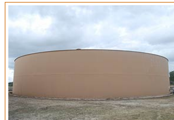
A job well done. Volunteers completed the big job in less than a day.
