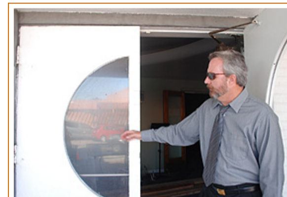
Michael McDermott, the City's Redevelopment and Economic Development Manager, inspects the door at the Perris Theatre. New doors will be installed as part of exterior renovations.
