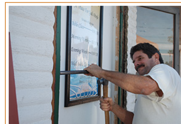
Craig Skrede removes stucco during the opening phase of exterior renovations.
