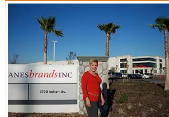
Associate Planner Diane Sbardellati outside the Hanebrands distribution center. The building will be honored April 28 as the largest green building in the world.
