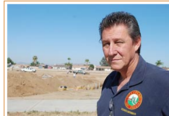
Perris City Councilman Mark Yarbrough looks over construction at Pinacate Middle School. The City and Perris Union High School District are working on a joint-use project at the site, which will include a gymnasium and classroom space.
