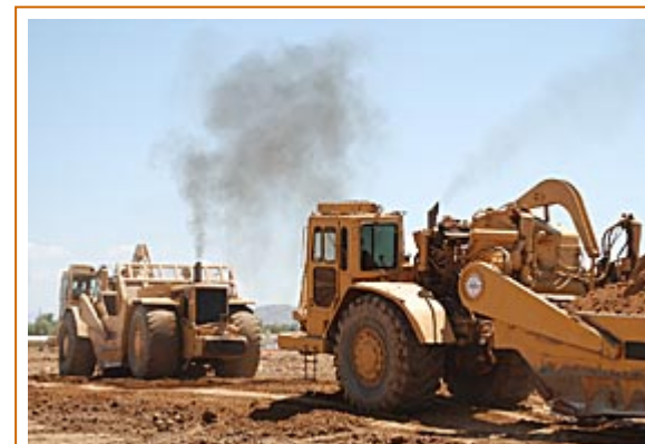
Giant earthmovers prepare the ground for the Field of Dreams.
