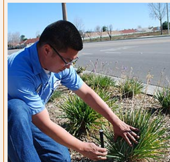
Perris Public Workers inspector Allen Yun examines a low-flow water sprinkler designed to reduce consumption at a City project on Placentia Avenue.
