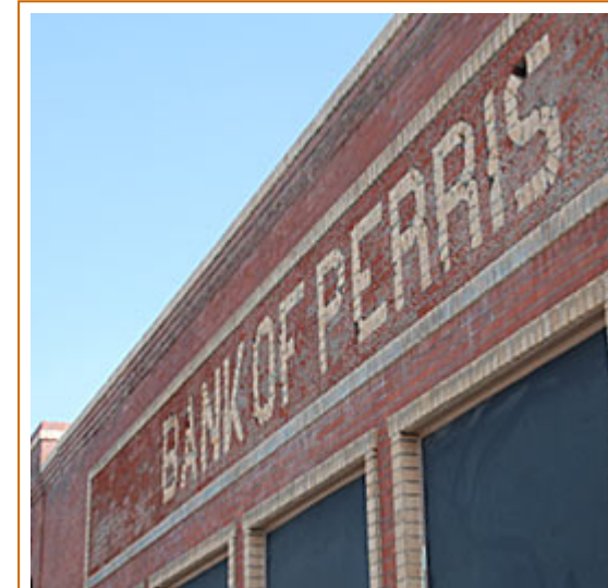
After applying a mild acid wash, the original letter of the Bank of Perris revealed itself after decades of being covered.
