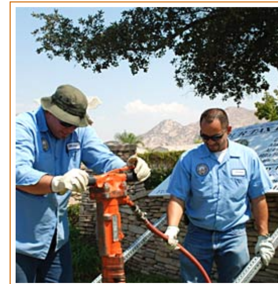
Workmen putting up a Slurry Seal project sign.
