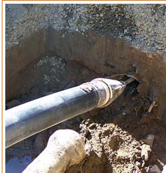
The pipe-bursting process in action.
