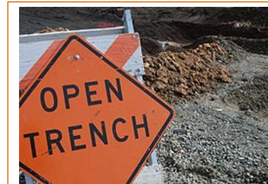
Warning signs dot the construction zone.
