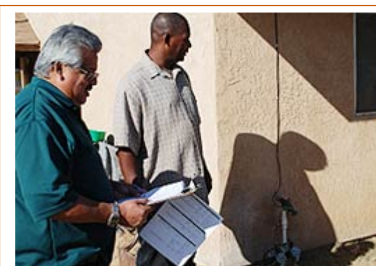
Gomez and McCarter inspect the sprinkler system, which could be replaced with grant funding from the Green Light for Savings Program.
