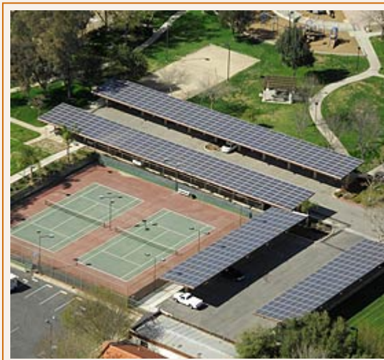
Aerial views of Perris solar-panel carports which were honored this week at the League of California Cities.
