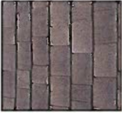
Clay Shingle Roof
