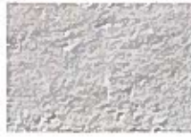
Painted Concrete Plaster Finish Color 1
