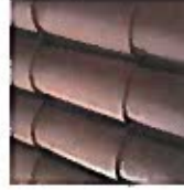
Clay Tile Roof
