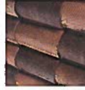
Clay Tile Roof
