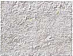
Painted Concrete Plaster Finish Color 1
