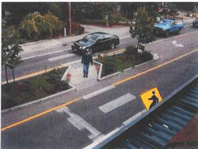
Figure 5: Median Island Pedestrian Refuge Crossing. Source: FHWA
