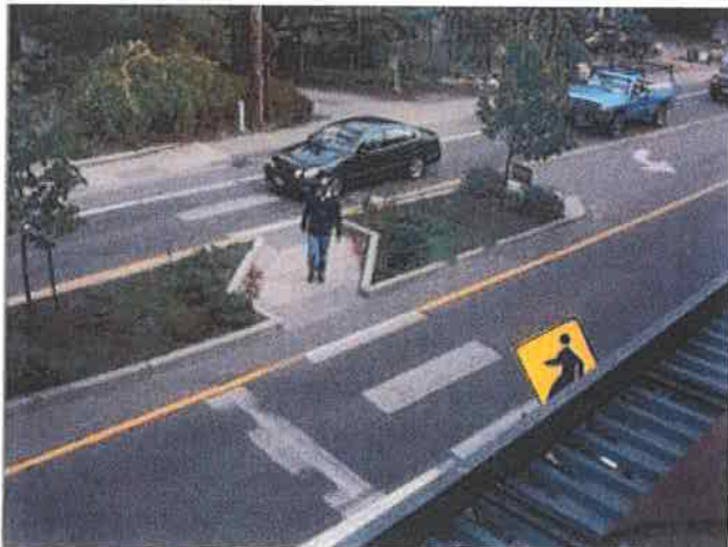
Figure 5: Median Island Pedestrian Refuge Crossing. Source: FHWA
