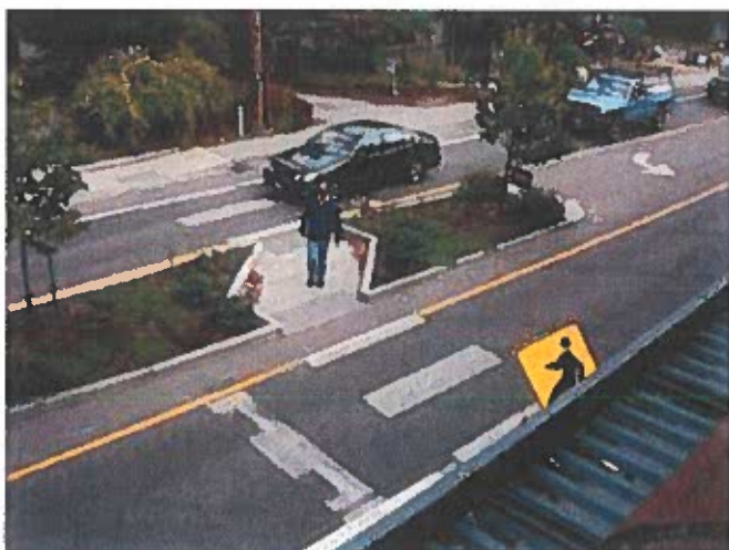
Figure 5: Median Island Pedestrian Refuge Crossing. Source: FHWA
