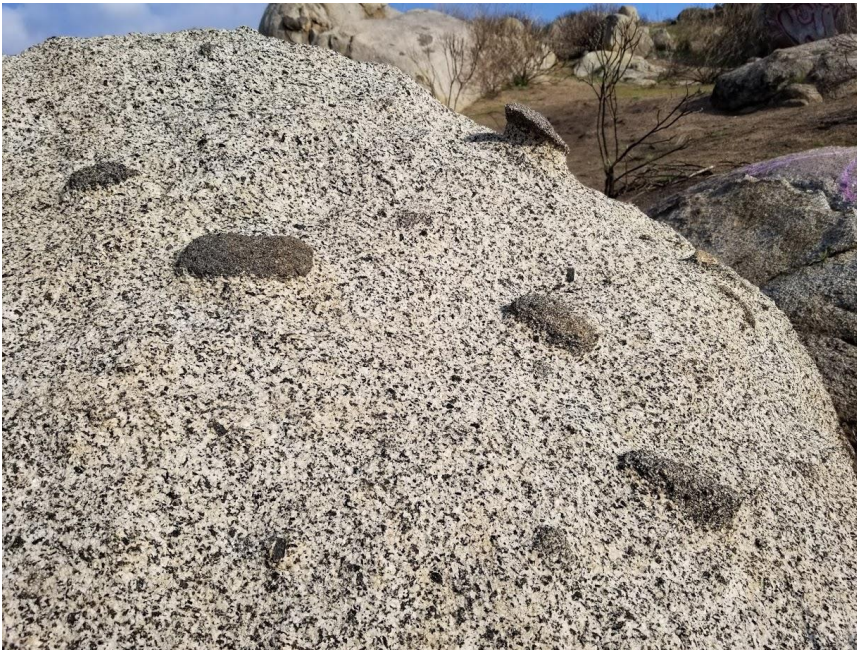
Photo 4: Exfoliated Granitic Boulder
