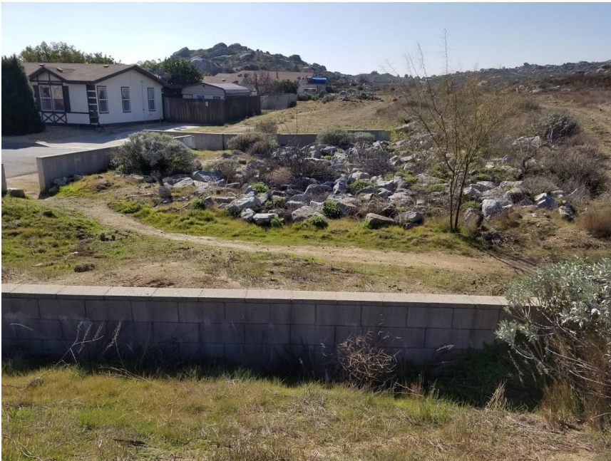
Photo 2: Project Overview Near Owl Drive Access Point (View South)
