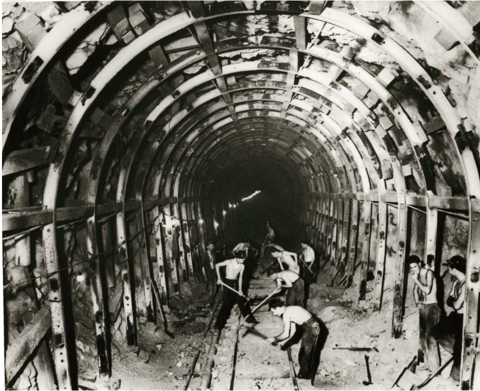
Figure 5. Workers in the Val Verde Tunnel, circa 1935 (Perris Valley Historical Museum).
