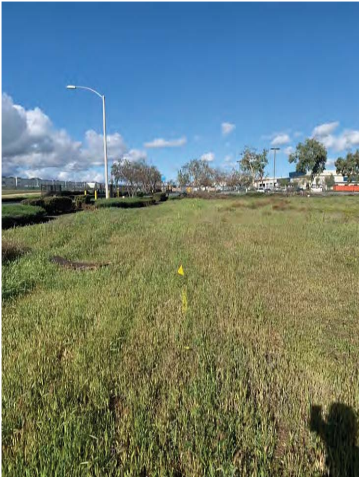
Gas Line Marked Out With Yellow Flags & Paint
