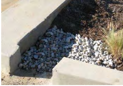
Figure 2: Curb Cut located in a Bioretention Facility
