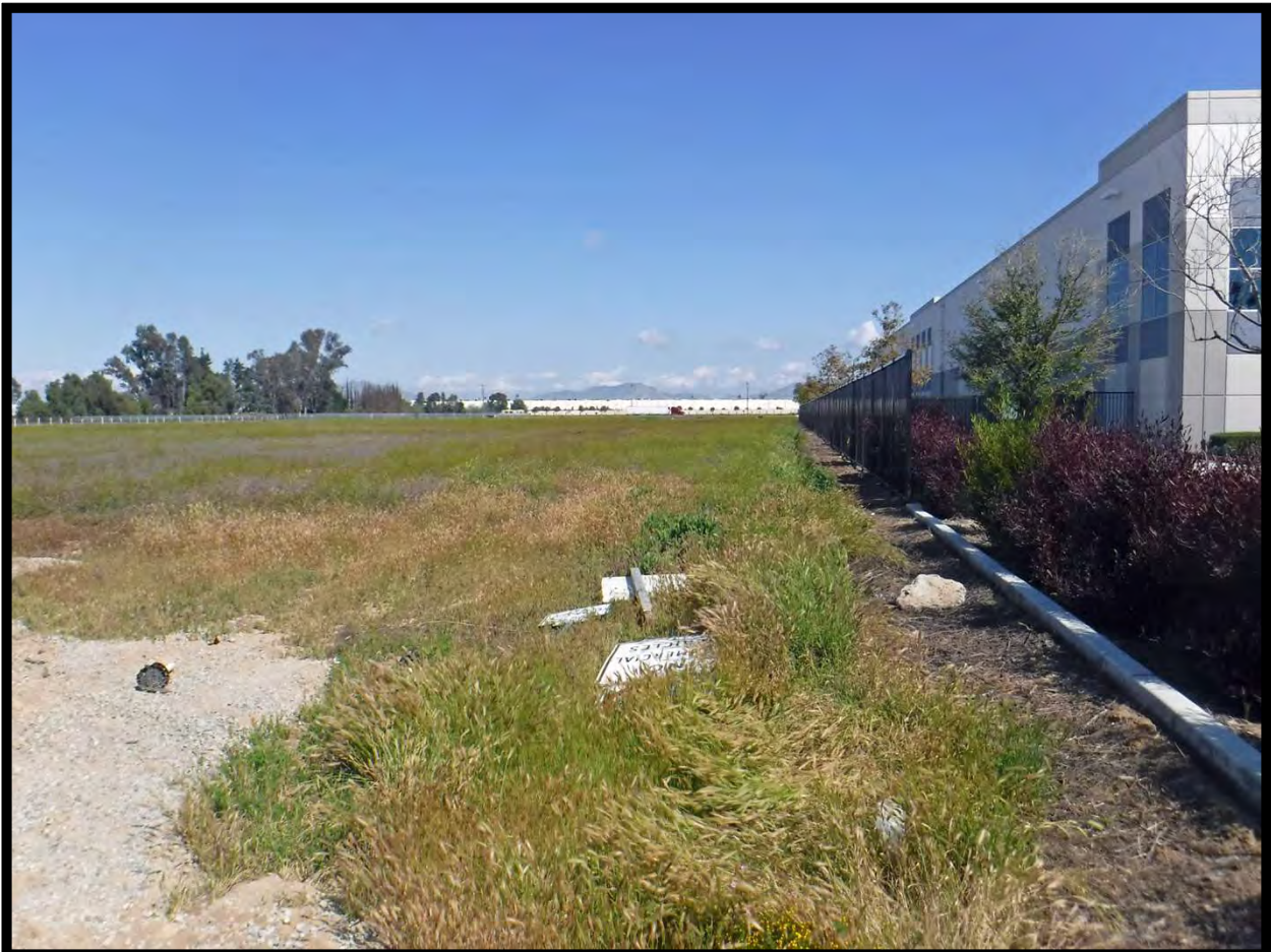
Overview of Eastern Property Boundary of Parcel -032 and Markham Street, Perris (N)
