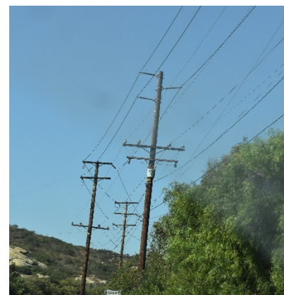
Example of overhead powerlines
