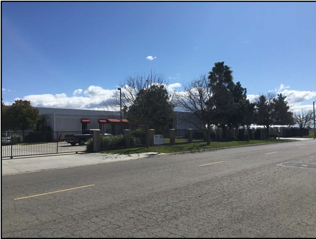
Plate 2: Overview of the previous development within the southwest quarter of the property, facing east across Wilson Avenue.
