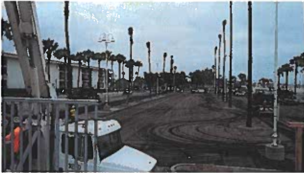
Belmont Pier Parking Under Construction
