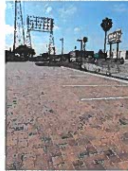
Redondo Beach Permeable Parking Lot
