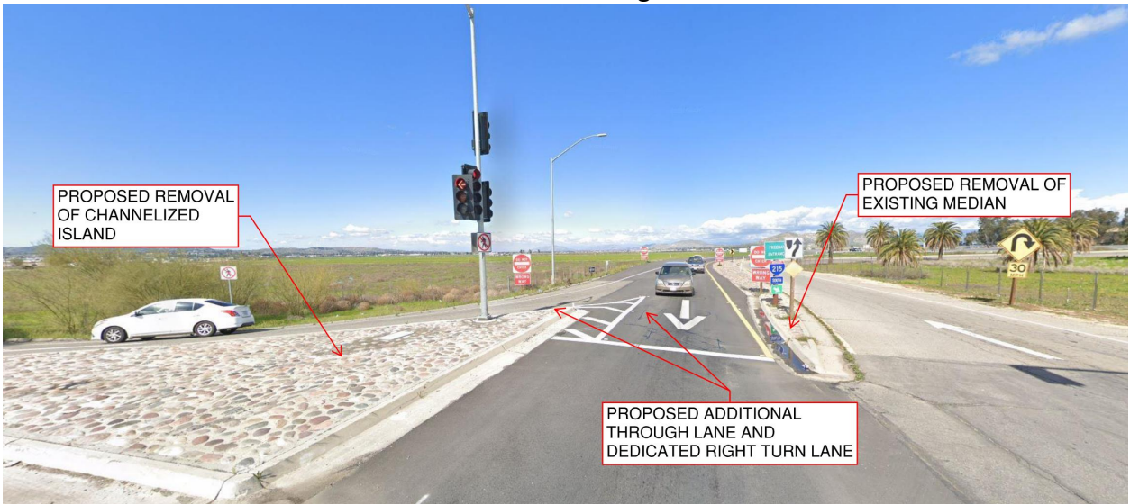
Photo location: I-215 Southbound Off-Ramp at Bonnie Drive Looking North
