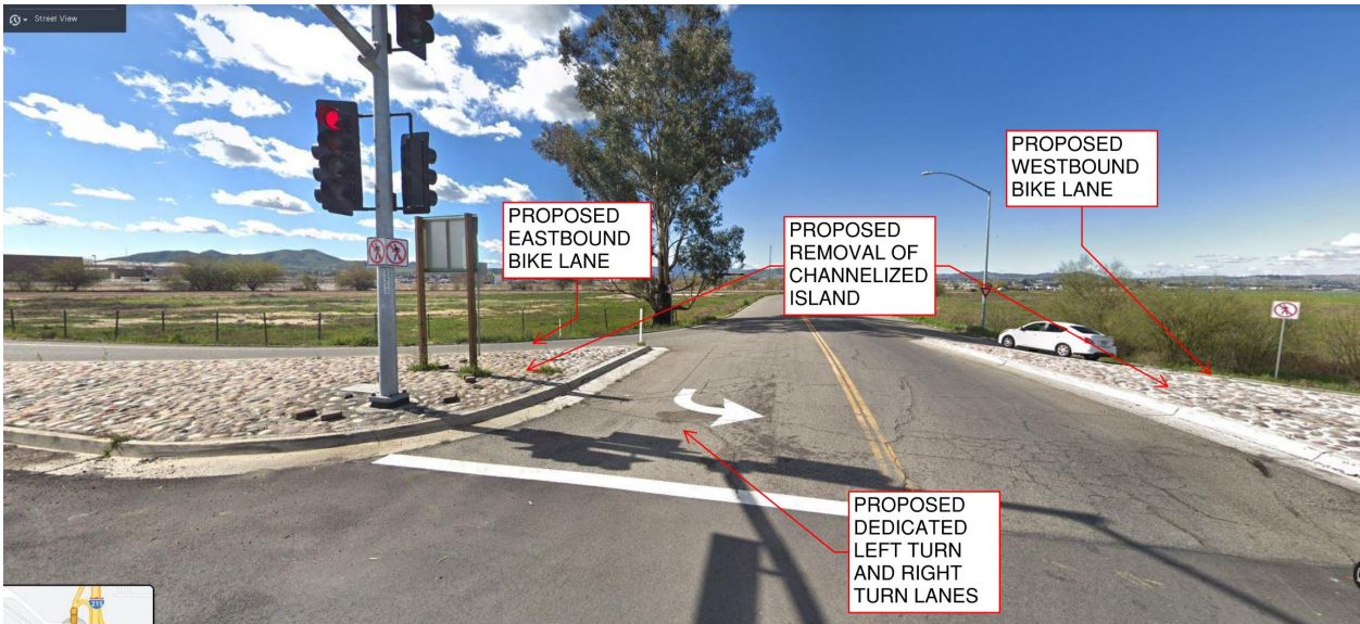
Photo location: Bonnie Drive at I-215 Southbound Ramps Looking West
