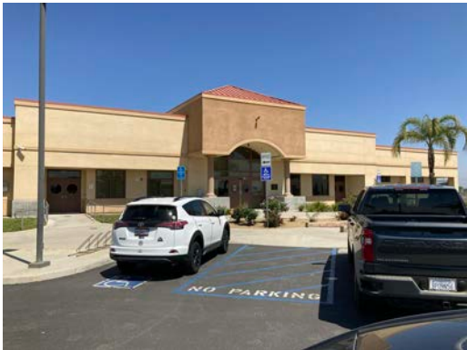
30. Adjacent to the south of Parcels 2, Val Verde Unified School District
