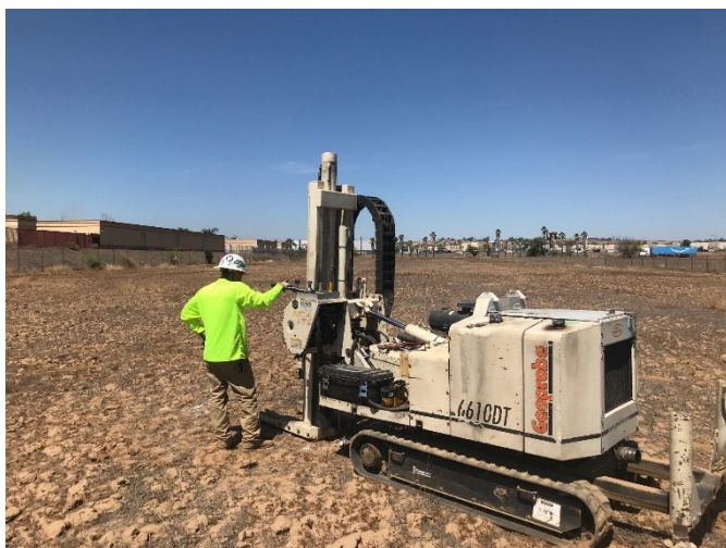
5. Geoprobe direct-push drilling rig set up at soil boring SB-3 in the southeastern portion of the Site
