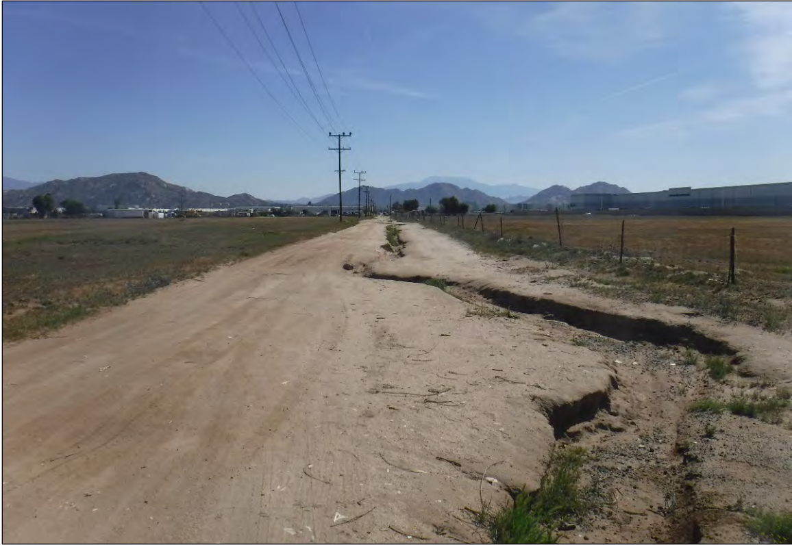
Figure 5-8 Looking east down West Nance Street.
