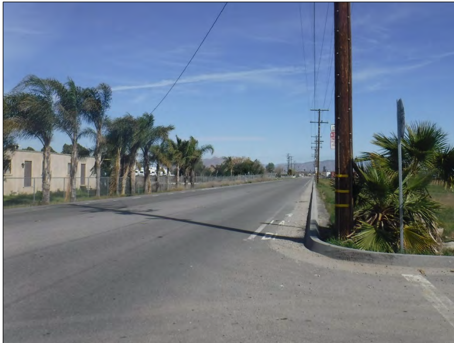
Photo 2: Patterson Avenue at intersection with Nance Street, looking north.
