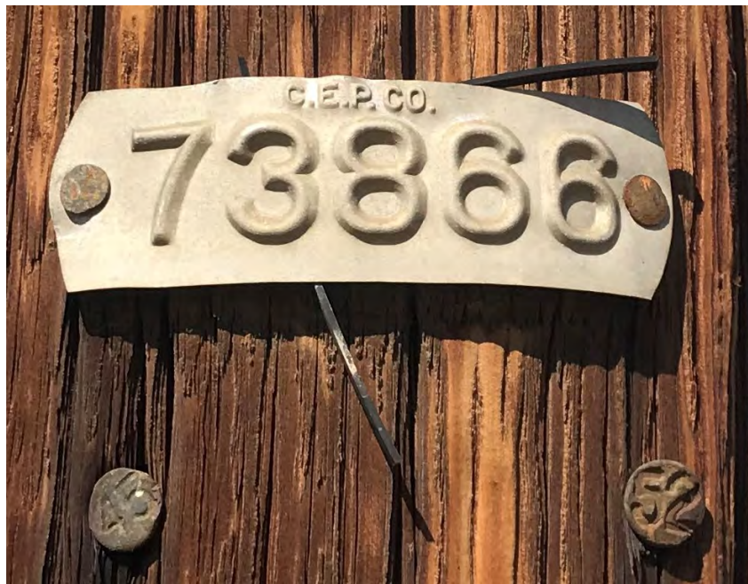
Photo 3: Date markers on one of the 11 poles along Nance Street.
