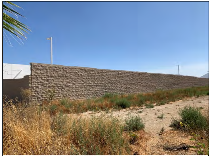
22. Adjacent property to the north from Ensenada Dr., view facing northeast.
