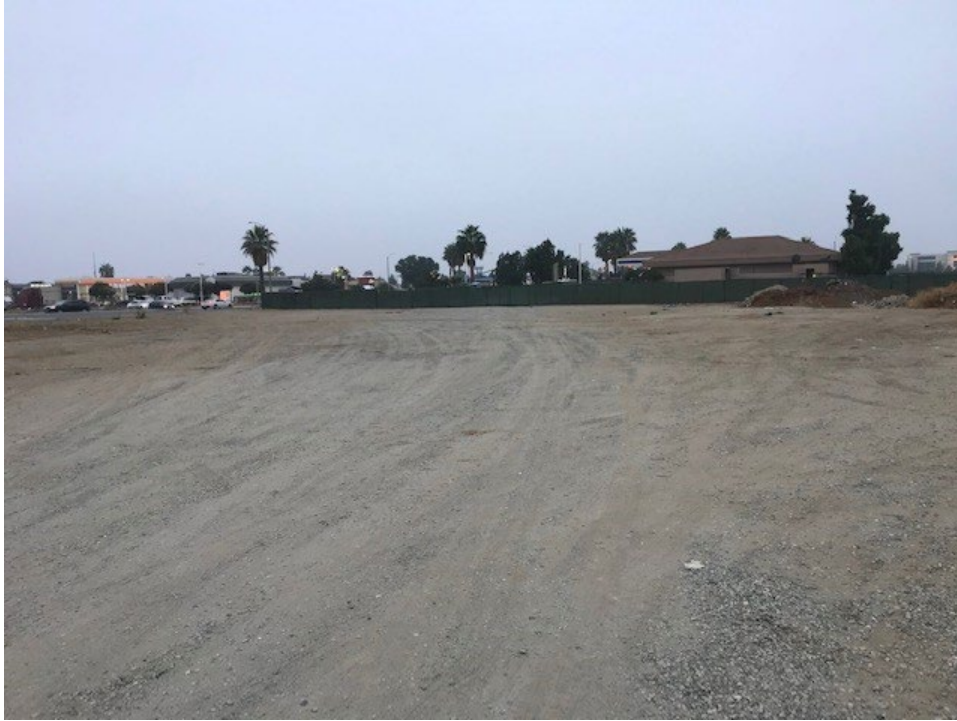
Plate 2. Graded area in the southeast corner of the project area, north of the gas station; view to the south.
