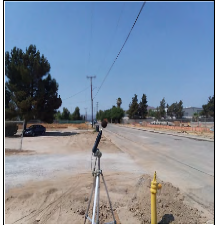
STNM4 looking NE up Wilson Avenue towards Rider Street intersection. Residence 3040 Wilson Avenue, Perris on the left.
