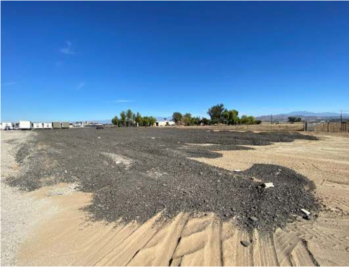
13. View of a typical area of imported asphalt-based placed in the northern and central portions of the Site, looking to the northeast.
