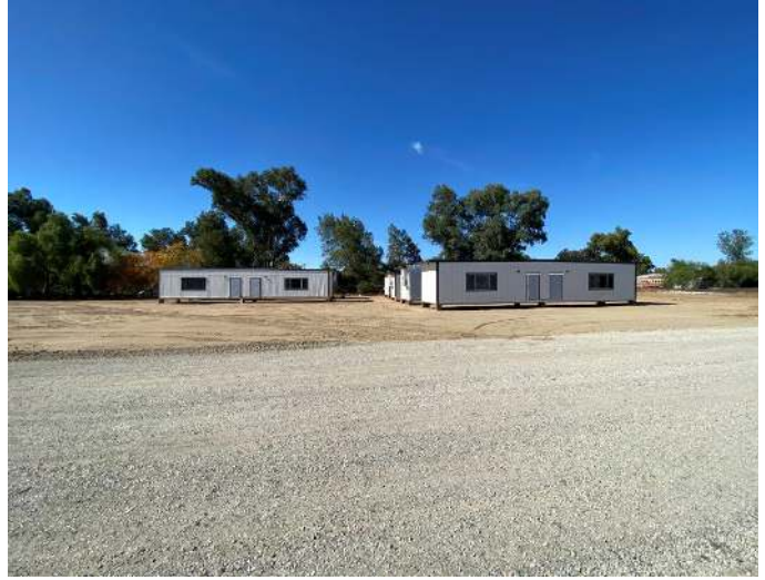
8. View of the office trailers/modular buildings stored in the southwestern portion of the Site, looking to the west.
