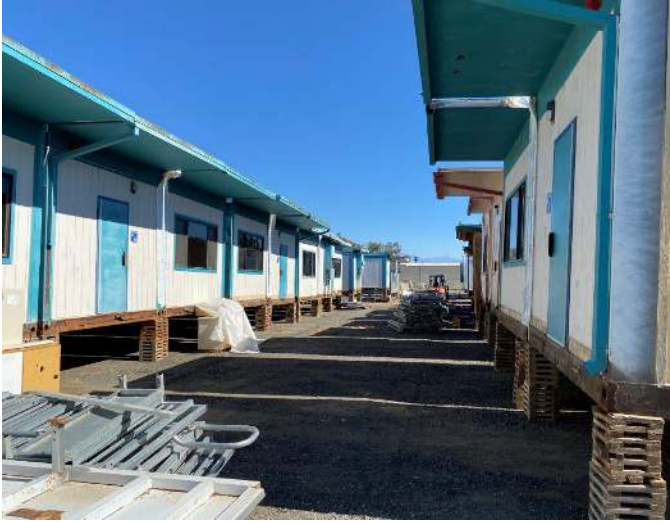
7. View of the office trailers/modular buildings stored in the northern portion of the Site, looking to the east.
