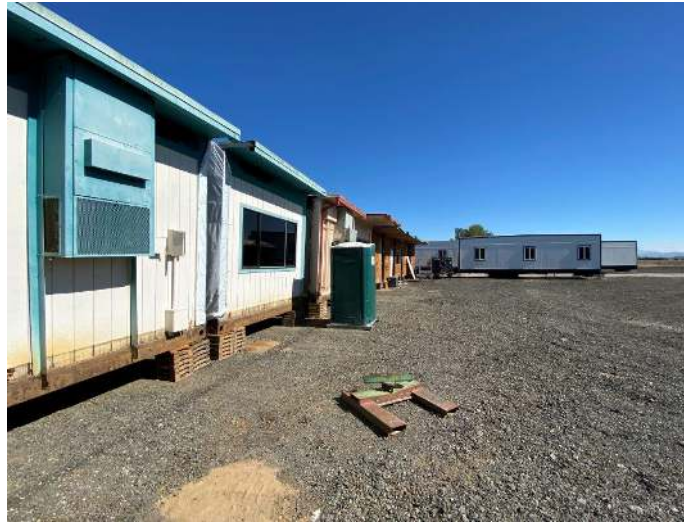
10. View of the office trailers/modular buildings stored in the northern portion of the Site, looking to the northeast.
