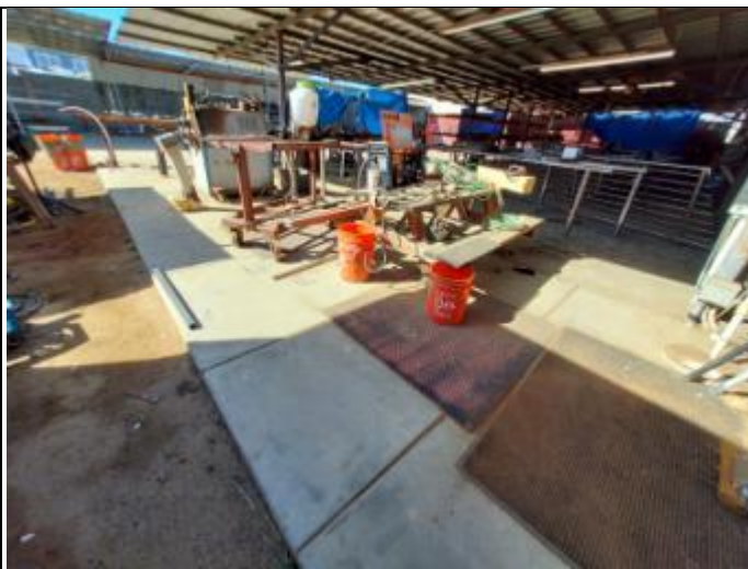
17. View of mobile office septic system cover 945 Markham.
